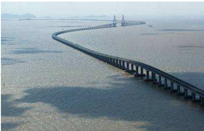
Dōnghǎi dàqiáo - 东海大桥 ( Shanghai ) – 32 km , 2005
