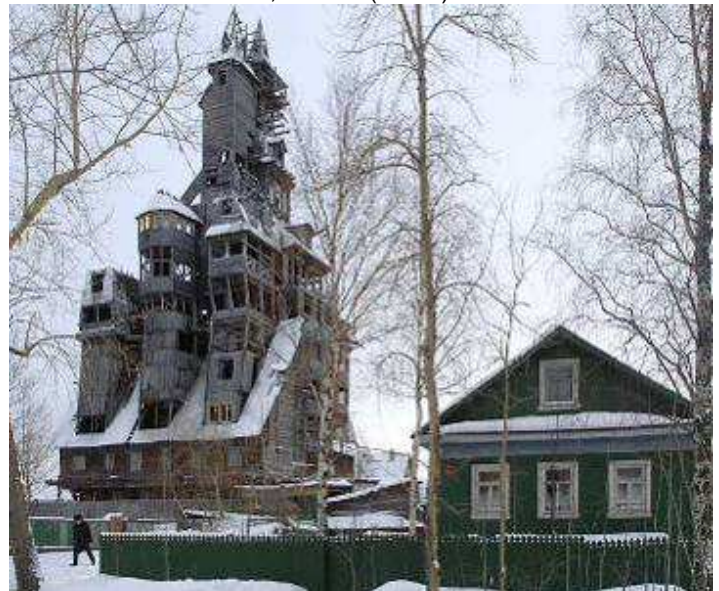
This wooden jumble of rooms and spires looks like it was built without the use of a spirit level. This was once the world's tallest wooden house, standing (just) in the Russian town of Arkhangelsk. Nikolai Sutyagin kept adding to the 12-storey house bit by bit, each time feeling that it still didn't look quite right. The house was demolished in 2008.
