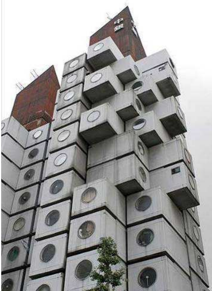
The Nagakin Capsule Tower,, Tokyo. 14 storeys. the 140 individual capsules were manufactured seperately and designed to be replacable.
