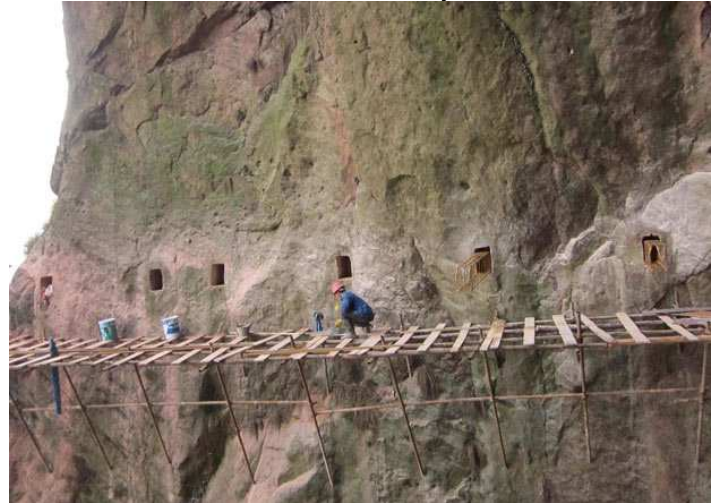
Building a plank road on Shifou Mountain is difficult because the cliff stands vertical at 90 degrees, without any slope or alcoves
